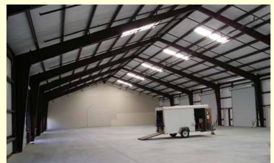
THIRTY FOOT INTERIOR ROOF LINE
